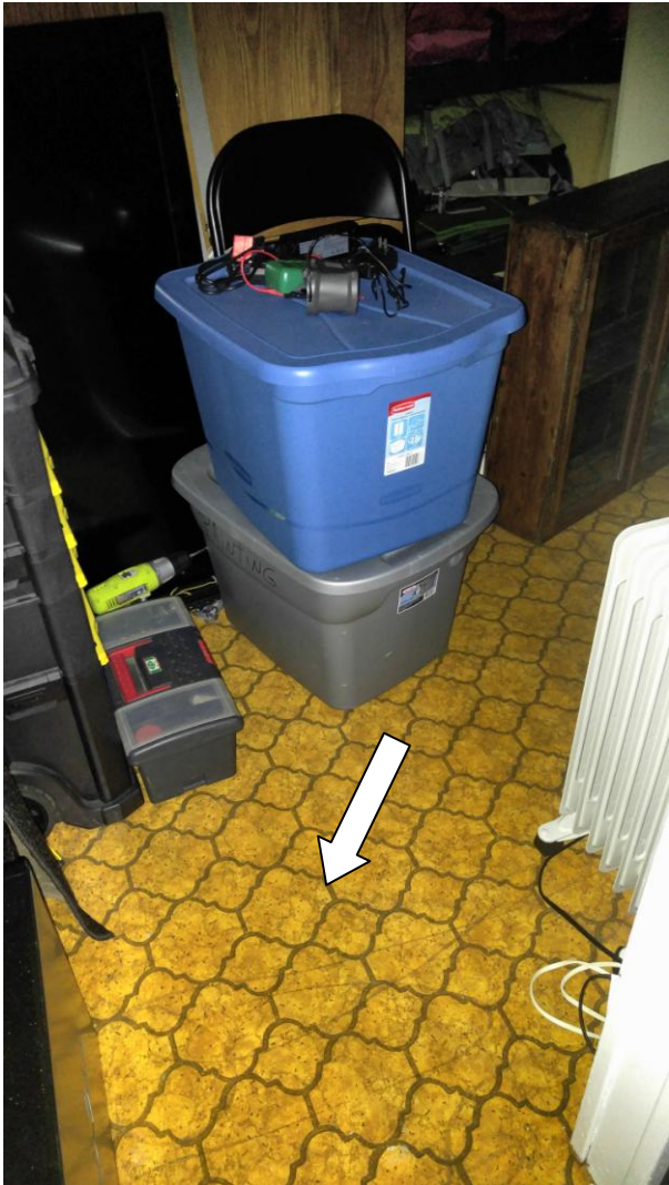
Asbestos containing Linoleum sheet flooring in the basement play room and asbestos containing Linoleum sheet flooring, drywall and ceiling texture in the kitchen of Unit 3036
