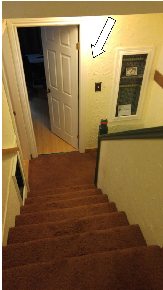
Non-asbestos containing wall texture on asbestos containing drywall in Unit 9042 and non-asbestos containing white and beige stucco outside Unit 9042
