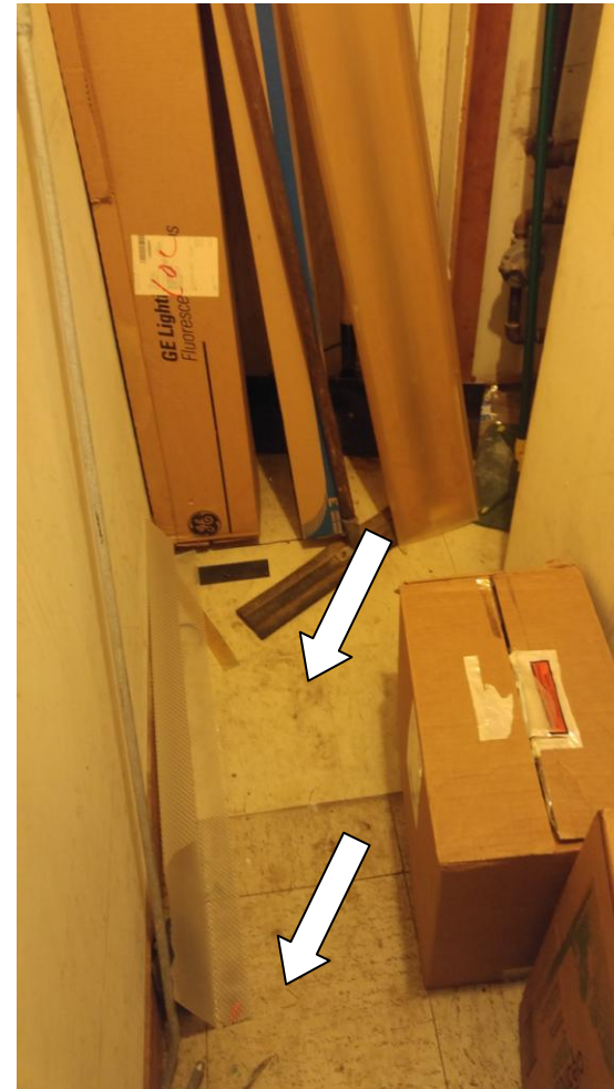
Asbestos containing red Linoleum in the basement of Unit 3051 and asbestos containing 12" white and grey vinyl floor tiles in the pool house janitor closet
