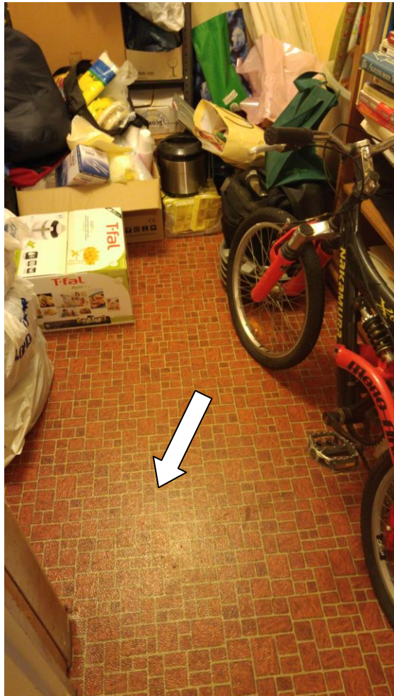
Asbestos containing red Linoleum in the basement of Unit 3051 and asbestos containing 12" white and grey vinyl floor tiles in the pool house janitor closet
