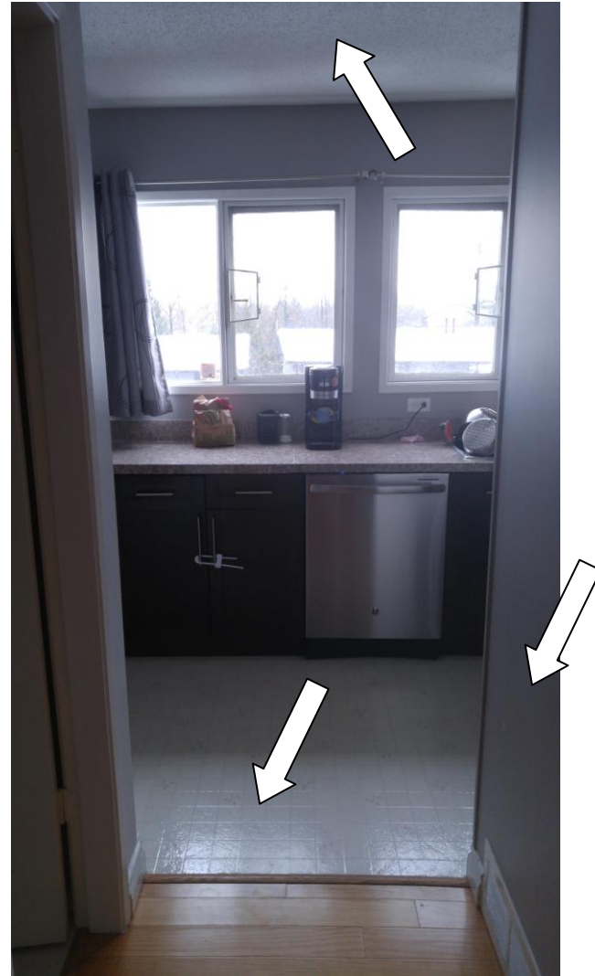
Asbestos containing Linoleum sheet flooring in the basement play room and asbestos containing Linoleum sheet flooring, drywall and ceiling texture in the kitchen of Unit 3036
